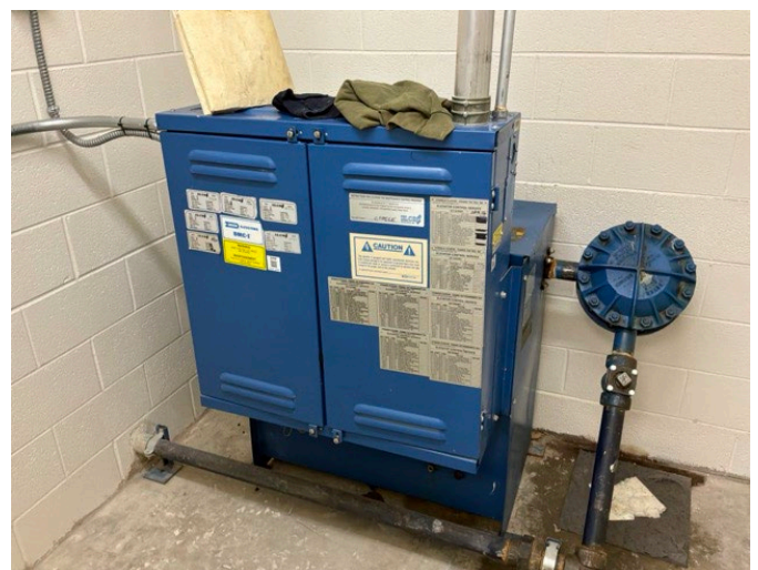
24 - ELEVATOR MACHINE ROOM
