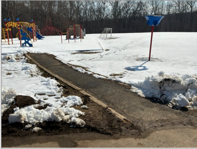
ACCESSIBLE ROUTE TO PLAYGROUND
