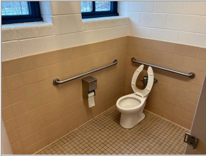
TOILET STALL OVERVIEW
